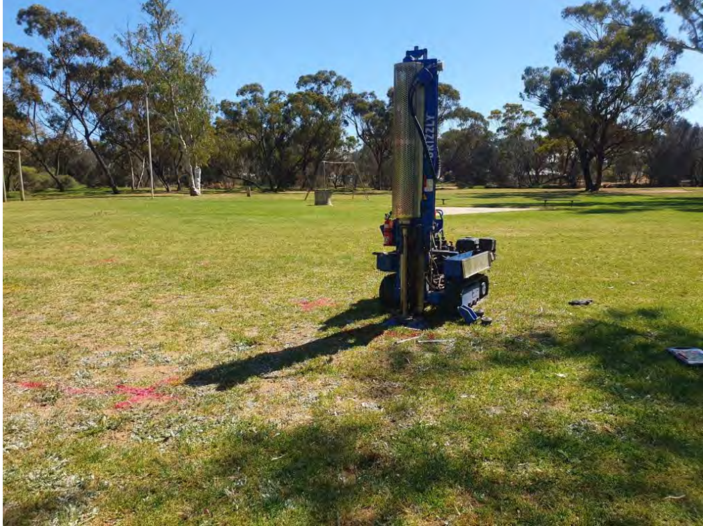
Photograph 3: Facing north, DPSH01 in progress
