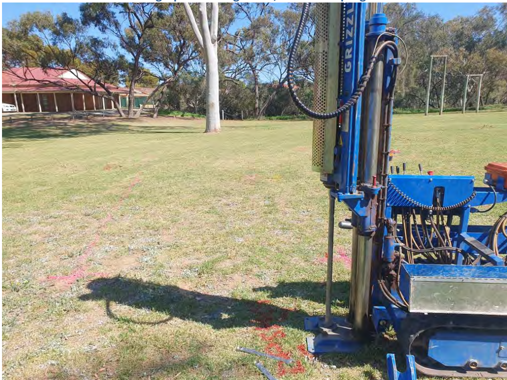
Photograph 4: Facing southwest, DPSH01 in progress
