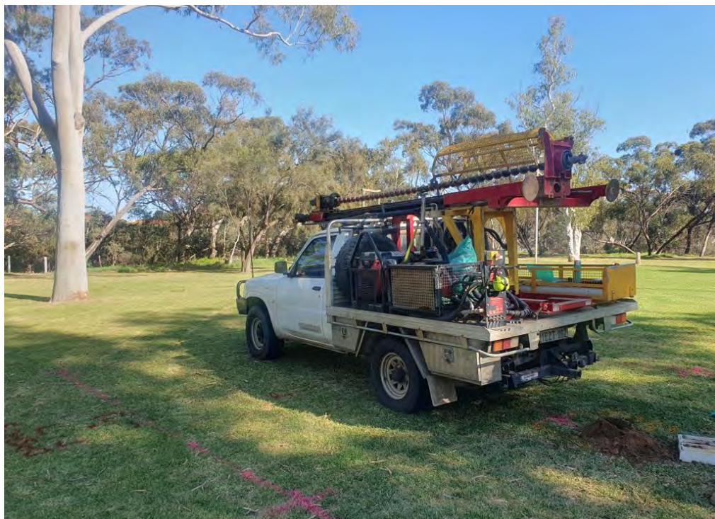
Photograph 2: Facing northwest at BH01 location
