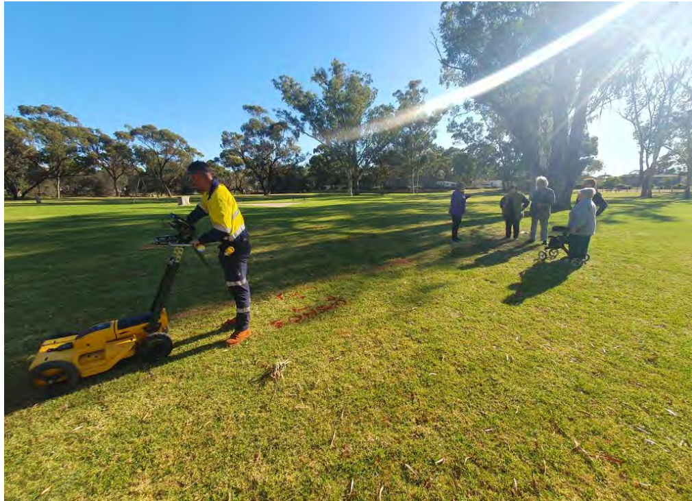
Photograph 1: Service location scanning carried out prior to works
